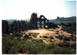
Photograph 3. The second tower for the Aspendos aqueduct has a 125 degree bend.
