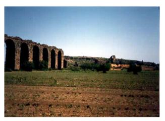
Photograph 2. To get across a valley, the Aspendos aqueduct used an inverted siphon carried on arches (venter). In the distance is the second tower.
