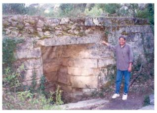
Photograph 3. The intake for the penstock at Jean de Mar Mill.
