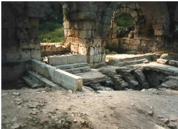
*Photograph 6. In this pool at the Southern Bath, Romans bathed in hot water. Note the underground central heating system.*
