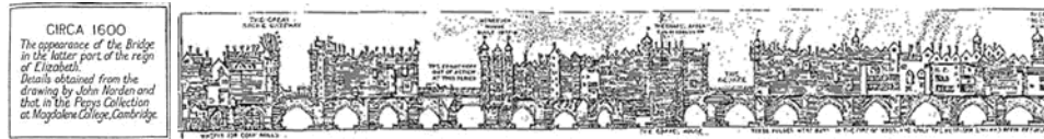
Figure 5. Artist's conception of London Bridge circa 1600. The first arch on the north was used for a water wheel and the first two arches on the south were occupied by wheels for corn mills (Home, 1931).
