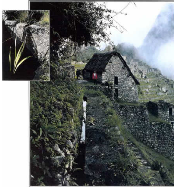
Photograph 2. The Inca supply canal flowed gently into Machu Picchu at an engineered grade on a carefully built terraced right-of-way.
