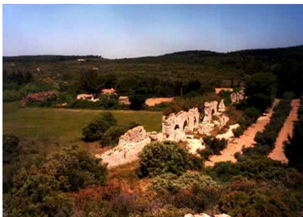
Photograph 4. This aqueduct provided water to a Roman mill at Barbegal and to the city of Arelate (modern-day Arles).
