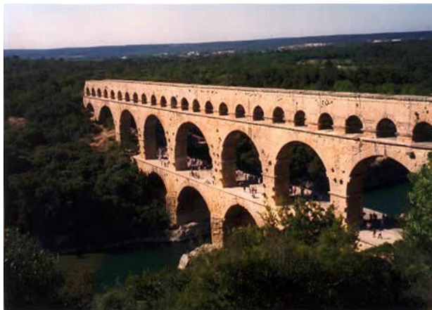
Photograph 1. Pont du Gard carried drinking water across the Gardon River Canyon to the ancient Roman community of Nemausus, modern-day Nimes.
