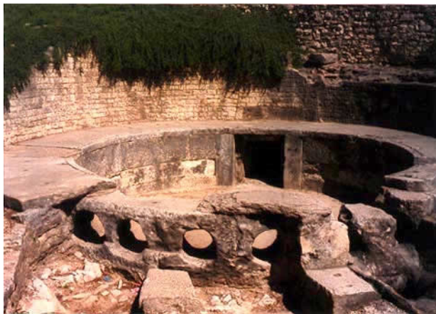
Photograph 3. This circular tank (castellum), located at the terminus of the Nemausus (modern-day Nimes) aqueduct. The holes were for lead pipes which distributed water throughout the city.
