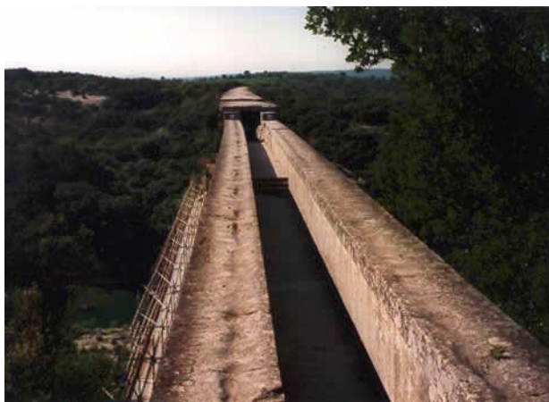
Photograph 2. The water channel on top of Pont du Gard was covered to prevent contamination and solar heating.
